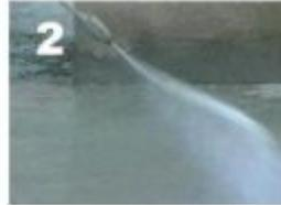
Remove from the surface dust, dirt, oil products, laitance, leach, shotcrete, plaster layers, tiles, paint and other materials that may impair penetration of the active chemicals contained in
